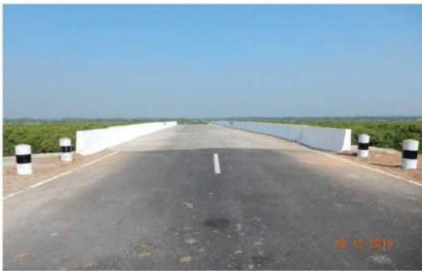
Figure 1: Bridge at Narayanapuram, Andhra Pradesh
