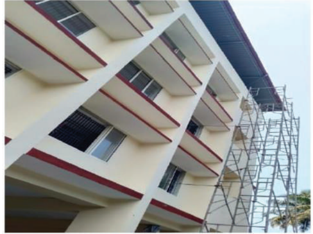
Figure 8: MPCS at Hosebette, Karnataka
