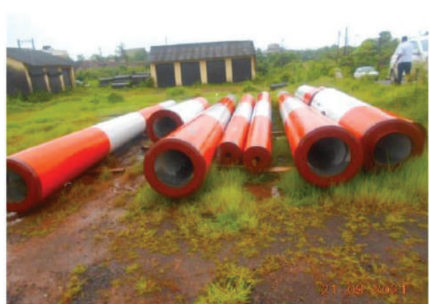
Figure 14: Spun tower of EWDS at MPCs, Goa
