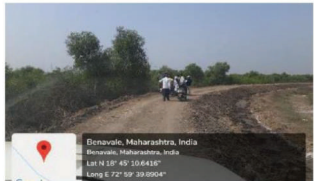
Figure 4: SE work under progress at Benavale, Maharashtra
