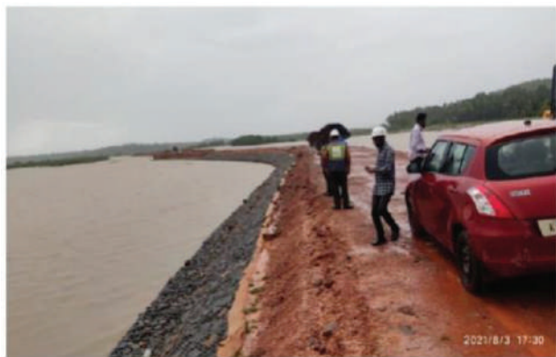
Figure 5: SE work under progress at Manikatta, Karnataka
