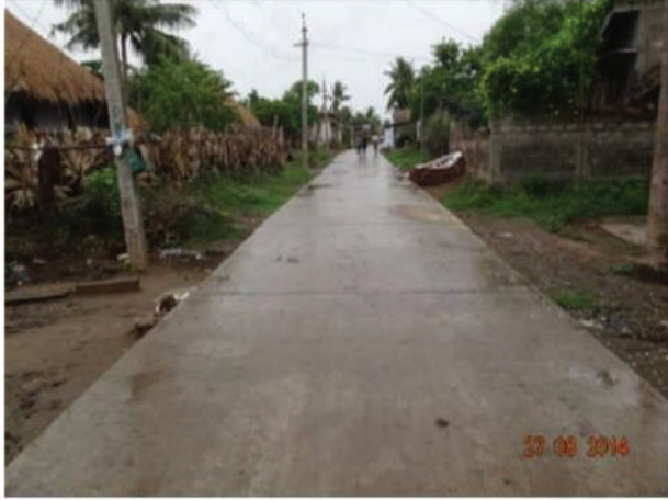
Figure 5: Road at Dindi, Andhra Pradesh
