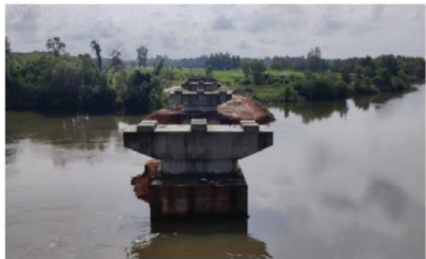
Figure 6: Bridge work under progress at Udpi, Karnataka
