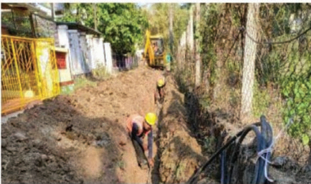
Figure 3: UGC work under progress at Alibag, Maharashtra
