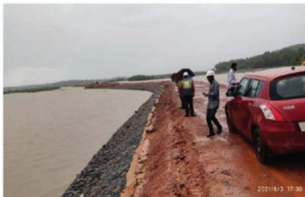
Figure 5: SE work under progress at Manikatta, Karnataka
