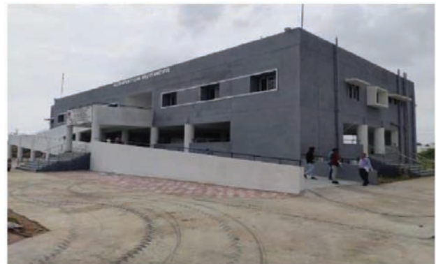
Figure 2: MPCS at Maktupur, Gujarat
