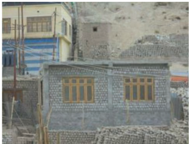
RC frame buildings with concrete blocks infill
