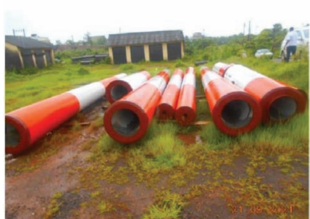
Figure 14: Spun tower of EWDS at MPCs, Goa
