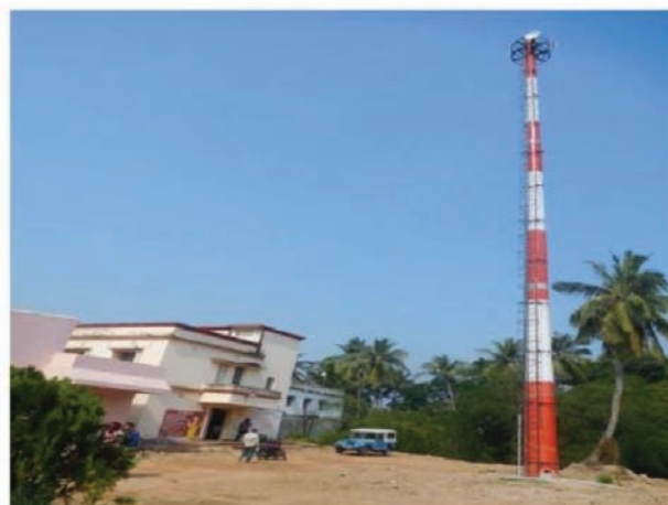
Figure 6: EWDS (Alert Siren) at Basudevapur, Odisha
