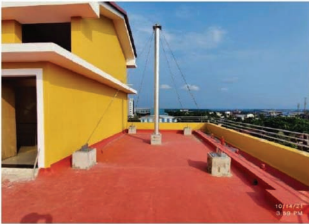
Figure 13: Mono pole tower of EWDS at MPCs, Goa
