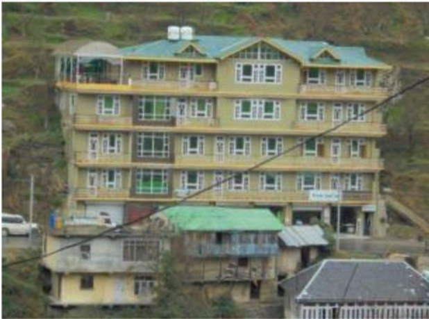
RCC Building with masonry infill
