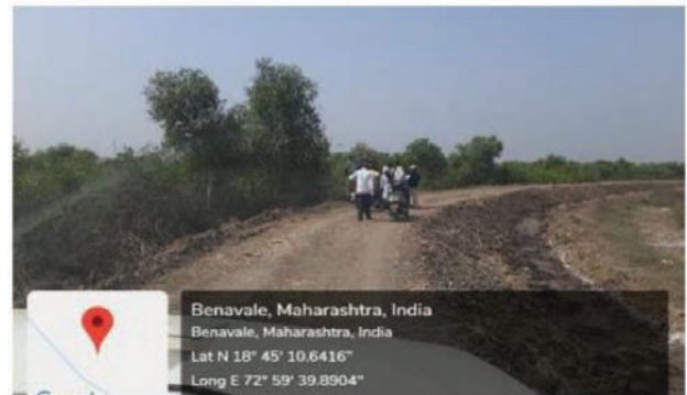
Figure 4: SE work under progress at Benavale, Maharashtra
