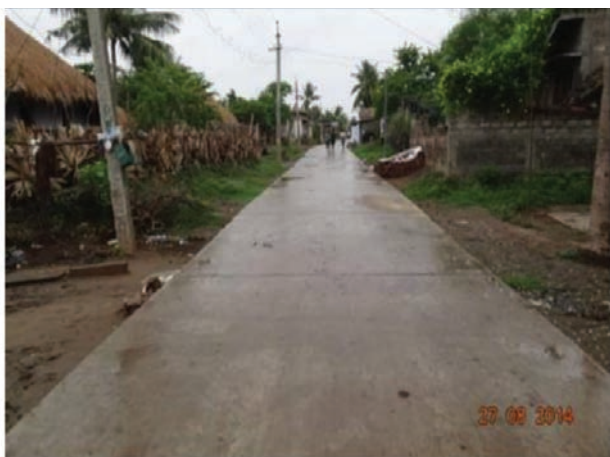
Figure 5: Road at Dindi, Andhra Pradesh
