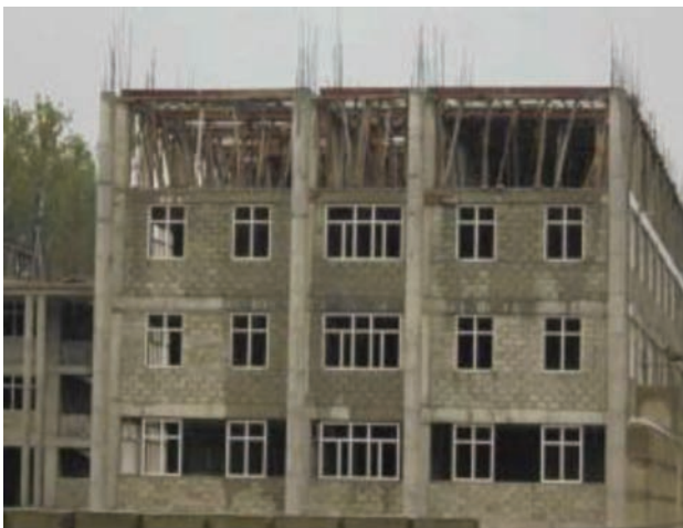
RC frame buildings with concrete blocks infill
