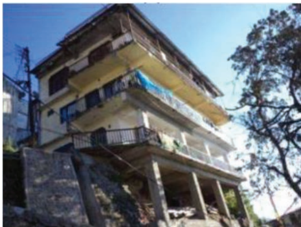
Contemporary buildings with retaining system and supported on stilts
