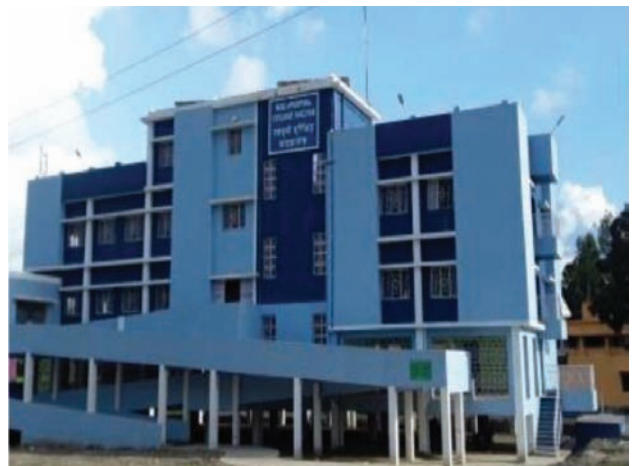
Figure 10: MPCS at Taranagar, West Bengal
