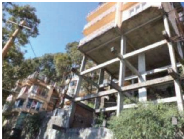
Contemporary buildings with retaining system and supported on stilts
