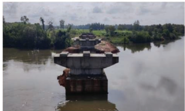
Figure 6: Bridge work under progress at Udpi, Karnataka
