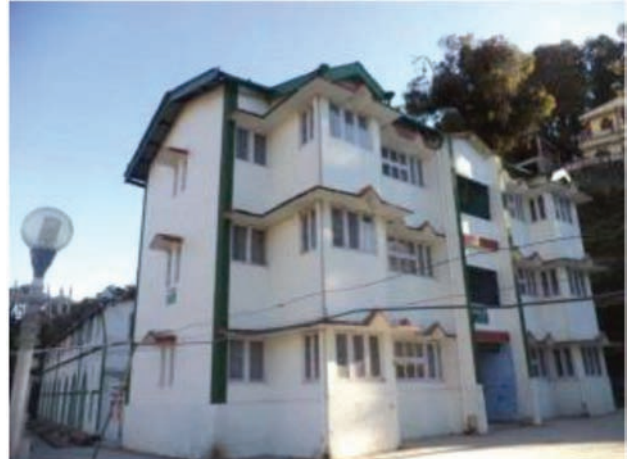
Burnt-clay brick masonry building
