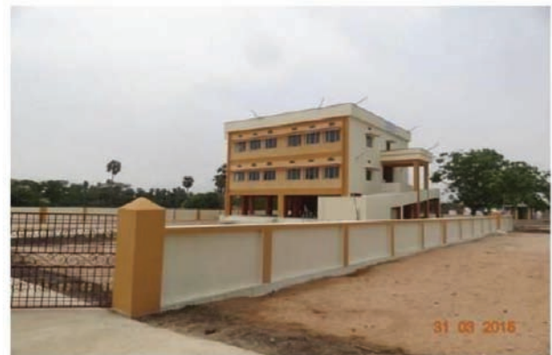
Figure 12: MPCs at Solmon, Andhra Pradesh
