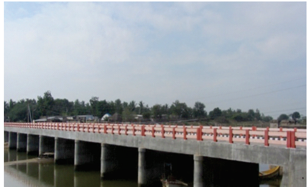
Bridge in Guntur District
