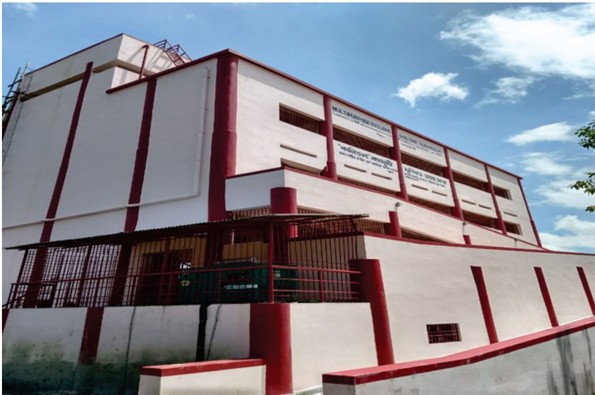
Construction of Cyclone Shelter at Haridashkati in North 24 Parganas District
